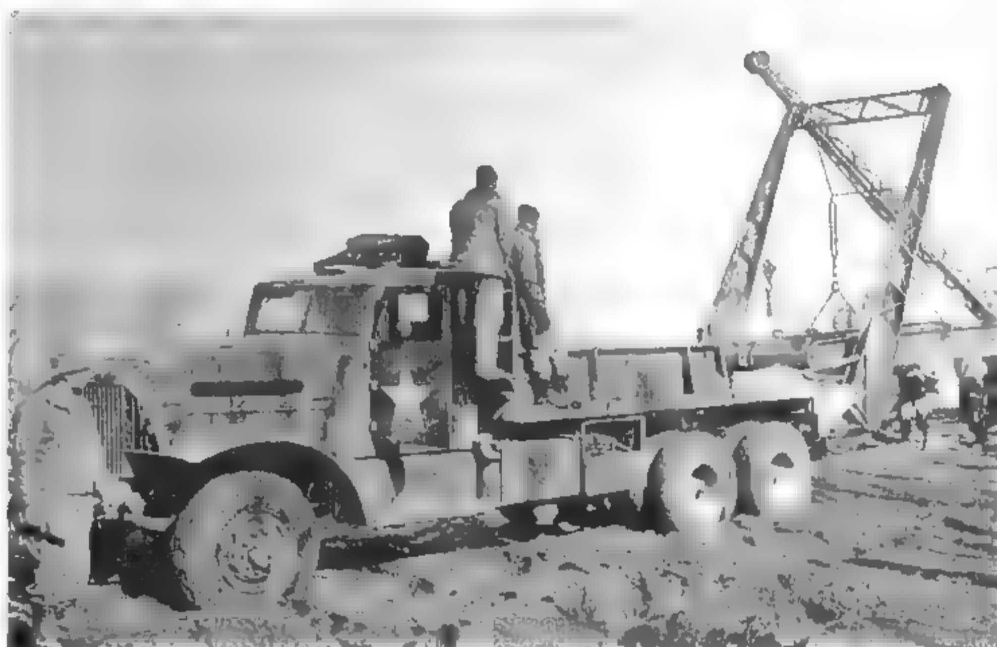
The hoist of this truck is being used to unload panels of a treadway bridge section. The bridge trucks were built on specially reinforced 220-in.-wheelbase chassis. (National Archives and Records Administration photo)
